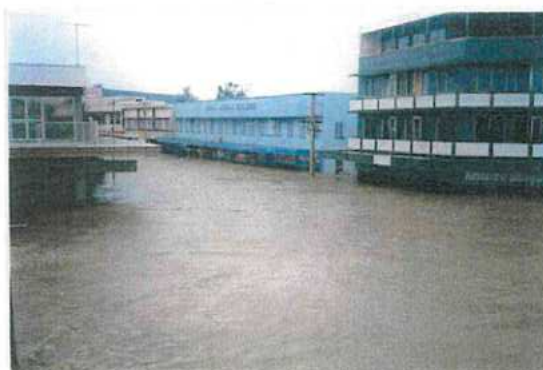
Flood in Nadi Town, April 2012
